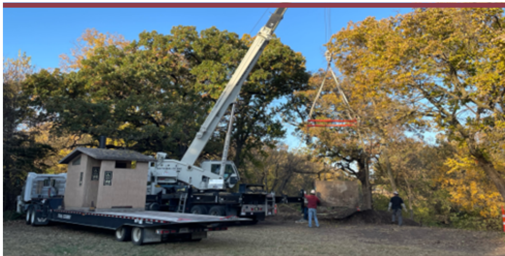
Photo: CXT & vault being loaded.
