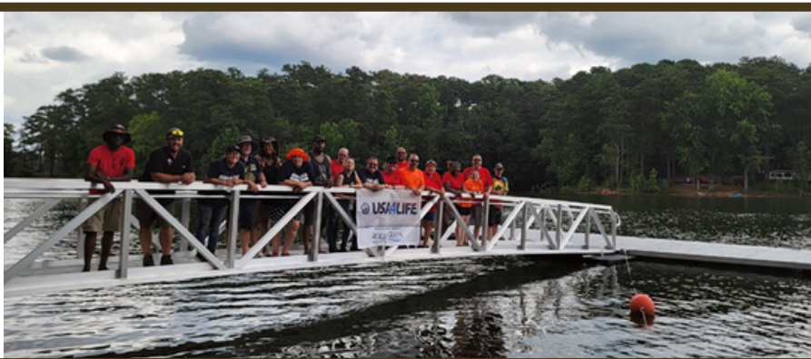
Above: Union Sportsmen's Alliance volunteers from SMART Local 85 and IBEW Local 613 standing on the newly installed AccuDock gangway at Allatoona Lake.
