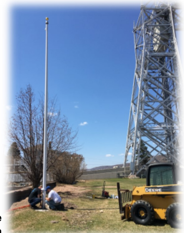
Signal flagpole installation
