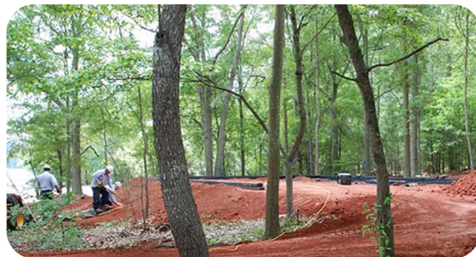
Crews work to construct handicapped accessible site at Coneross Campground.
