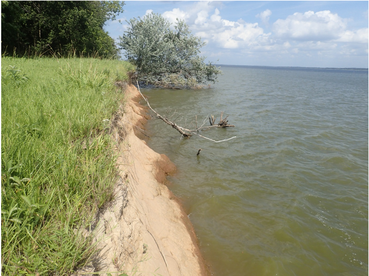
Photo of existing shoreline erosion (north view)
