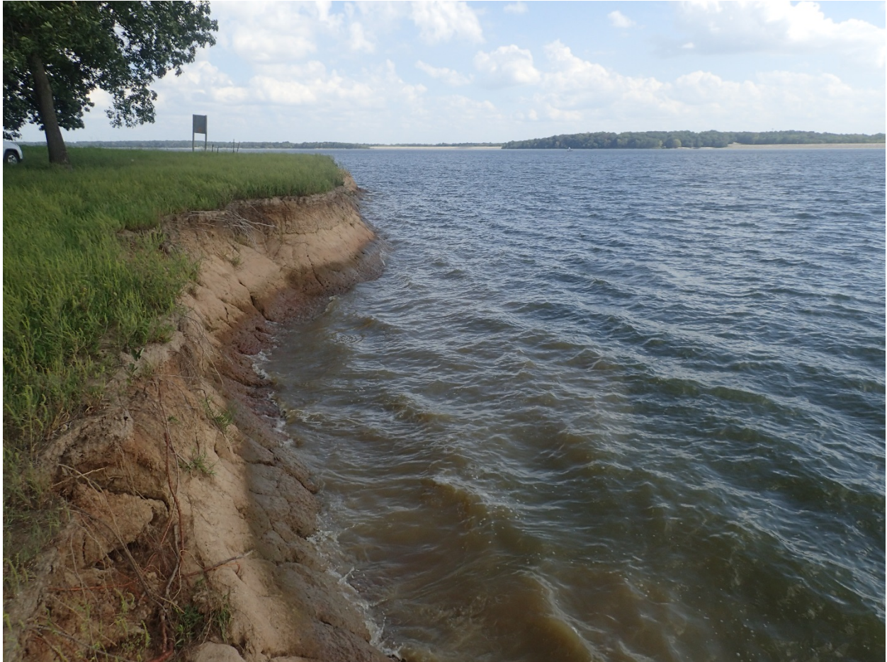
Photo of existing shoreline erosion (west to east view)
