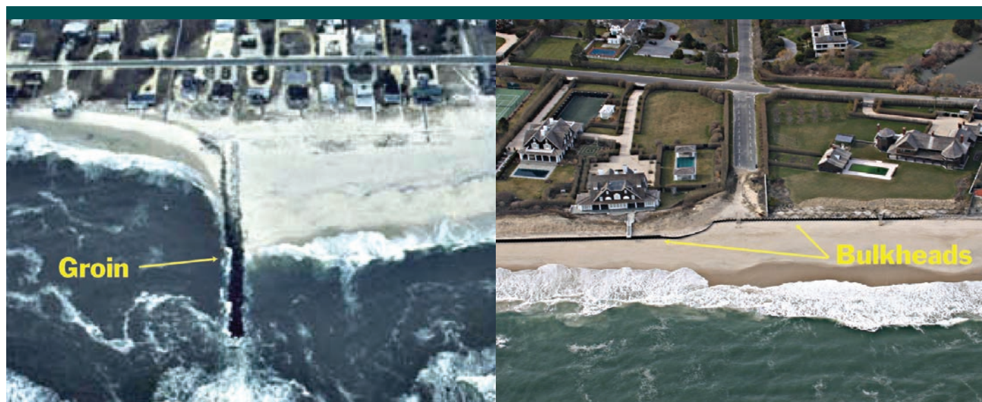
Figure 22. The most commonly used erosion control structures on the south shore are shore perpendicular structures like the groin on left and shore parallel structures like the bulkheads on right. (Bulkhead photo: First Coastal Corp)
