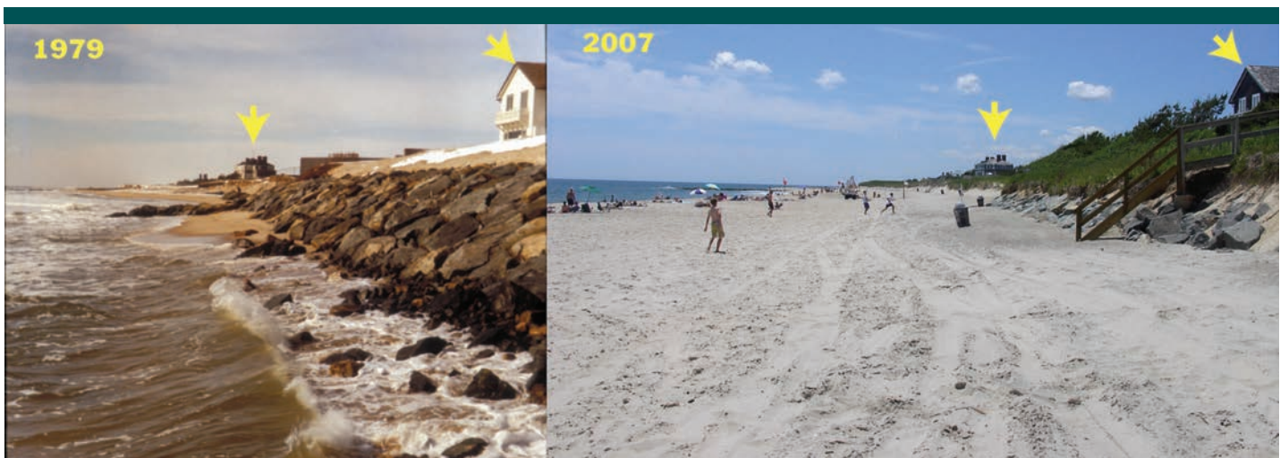
Figure 24. In stable areas with an adequate sand supply, studies over the last thirty years have shown shore parallel structures like this rock revetment can provide erosion protection during severe storms without adversely affecting natural beach building processes. (Arrows indicate the same houses in the two photos for reference.) (2007 Photo: M. Slattery)
