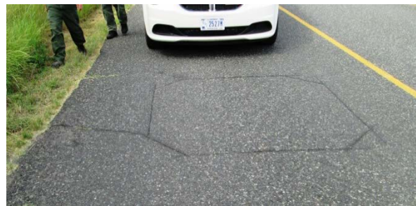
Figure 22 - Example of a properly cut single-lane loop
