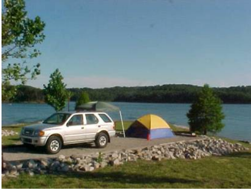
Figure 1. Typical hardened pad provided for COE campsites and picnic areas, with a fine crushed stone surface. This campsite at Moutardier Campground, Nolin River Lake, KY also has a riprap border to prevent erosion when the lake level rises
