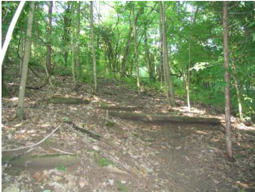
Figure 4. Taylorsville Lake, KY. This steep section of interpretive trail does not have erosion problems, but safety issues arise due to being very slick when wet. Installation of a hand rail is recommended.
