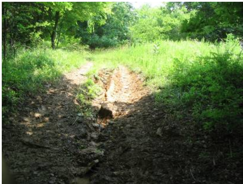
Figure 7. Taylorsville Lake, KY. Erosion on portion of the trails at Taylorsville Lake State Park, Possum Ridge area. This trail has been heavily impacted by horses.
