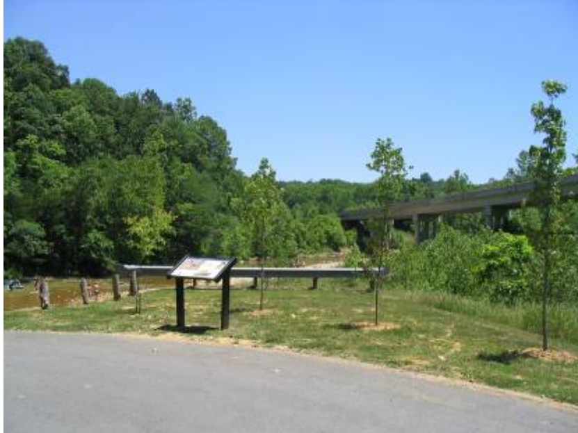
Figure 13. Otter Creek Park, KY. Small trees planted between the guardrail and the roadway have effectively stopped cars from pulling into the grassy area, where soil compaction and loss of vegetation due to the vehicles had been a problem
