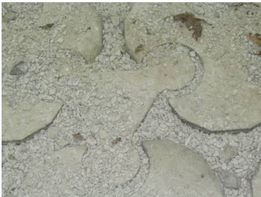
Figure 28. Cave Run Lake, KY. Close up view of Tri-lock block placed on the trail. “Tri-lock is a system of pre-cast concrete blocks made up of two components: a ‘lock block’ and a ‘key block’. Each is keyed into two other components for stability and integrity. For ease of installation, the blocks are typically installed in dry conditions by hand on a specially engineered filter fabric” (Hanson, )
