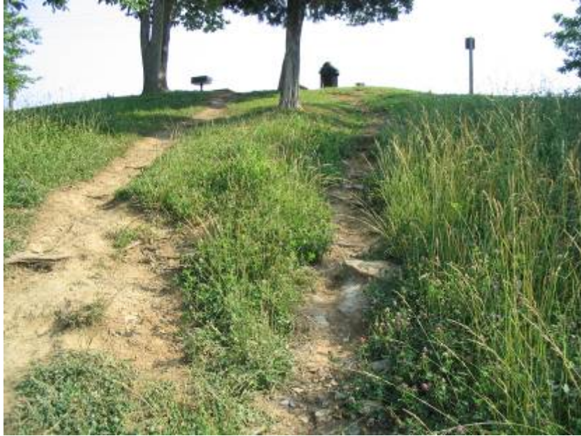
Figure 3. Taylorsville Lake, KY. Erosion on trail created by bank fishermen just upstream of the right abutment of Taylorsville dam.
