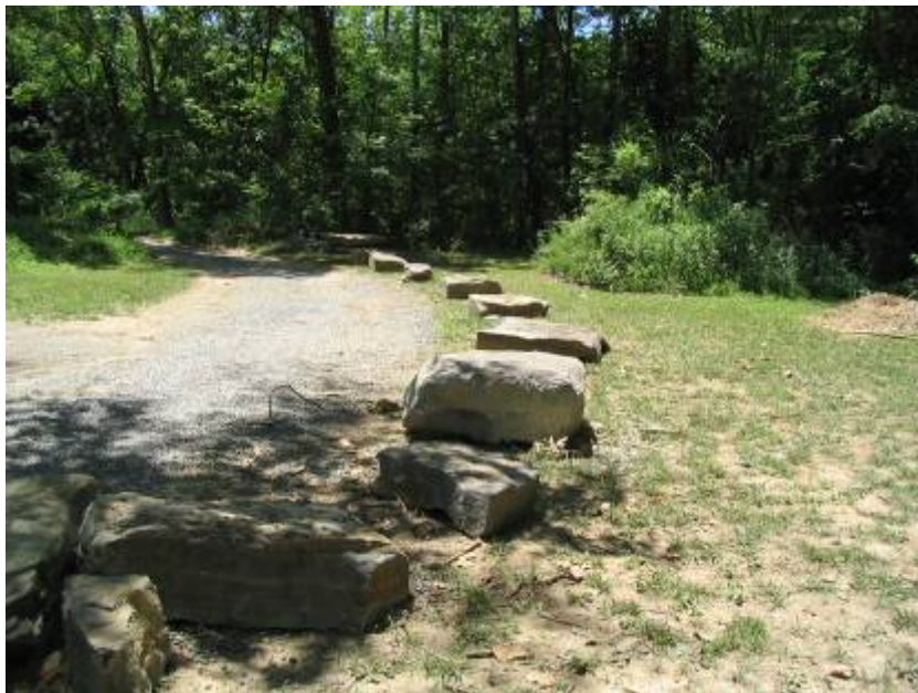
Figure 14. Otter Creek Park, KY. Large rocks from a nearby road cut used as natural barriers to keep vehicles out of the grassy picnic area
