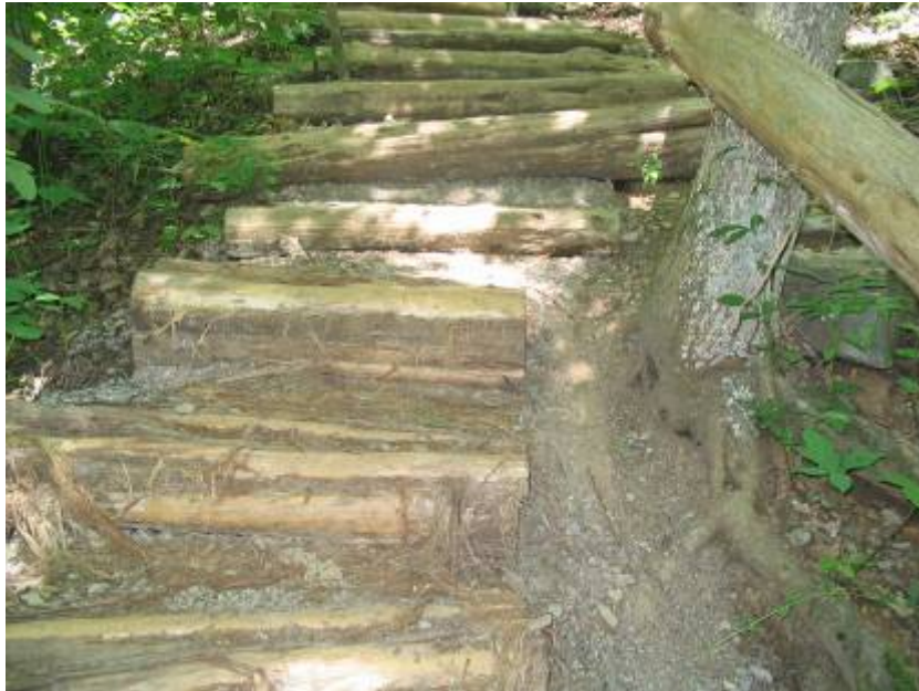
Figure 17. Otter Creek Park, KY. An old section of trail with steps made from cedar trees
