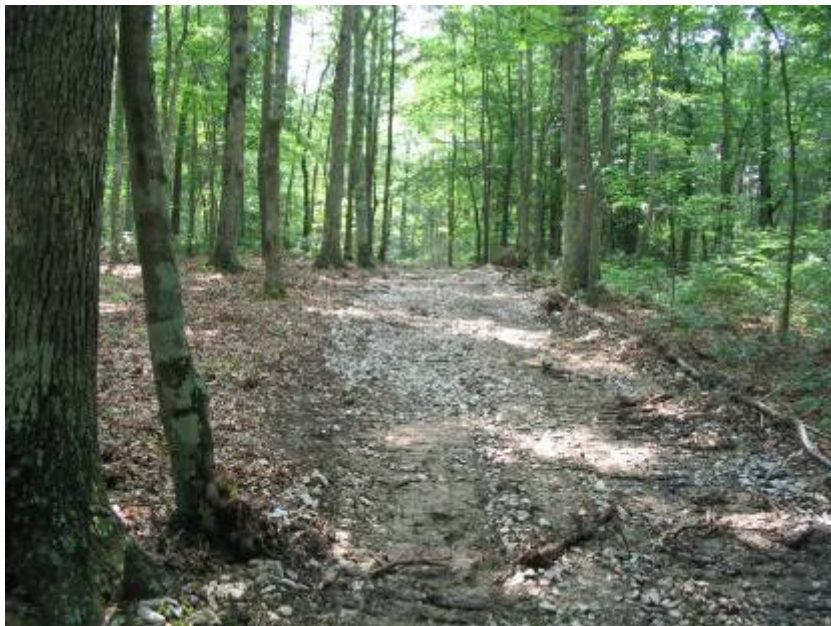
Figure 33. Cave Run Lake, KY. July 2005, Sheltowee Trace Trail rehabilitation. Note dozer tracks. Because hand labor is so slow and cost prohibitive, the USFS uses small dozer for initial construction and major trail rehab to clear and level trails. The addition of gravel to the tread gives an initial appearance of “a small road” in the word of USFS representative Loomis
