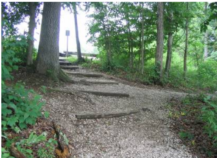
Figure 21. Cave Run Lake, KY. This trail to picnic sites in the COE's Stoney Cove Recreation Area utilizes timber water bars and gravel to slow erosion. Park Manager Barnum notes that "the selection of crushed stone sizes to harden problem areas along trails depends upon the gradient of the trail segment and underlying soils. Class I sand (limestone chips) is far superior as a walking surface (packs well, lays flat and is quiet); however, it is unsuitable as a hardening material along steeper sections of a trail. Larger stone, such as No. 57 or No. 610 are heavier and resist erosion better. But the angular pieces of larger stone do not pack well, are noisy to walk over and tend to roll under foot"
