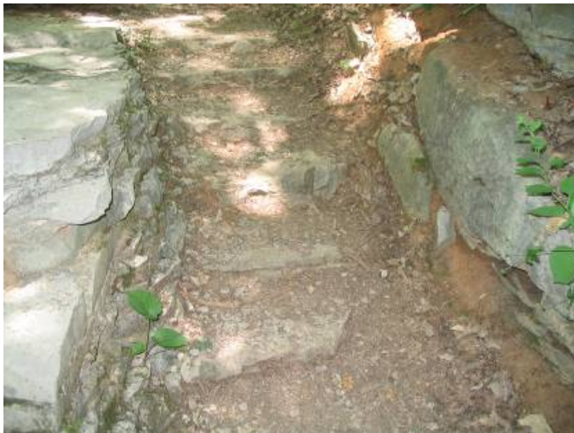
Figure 16. Otter Creek Park, KY. Steps on this section of trail were jack-hammered from an existing boulder in the trail's path about 15 years previously
