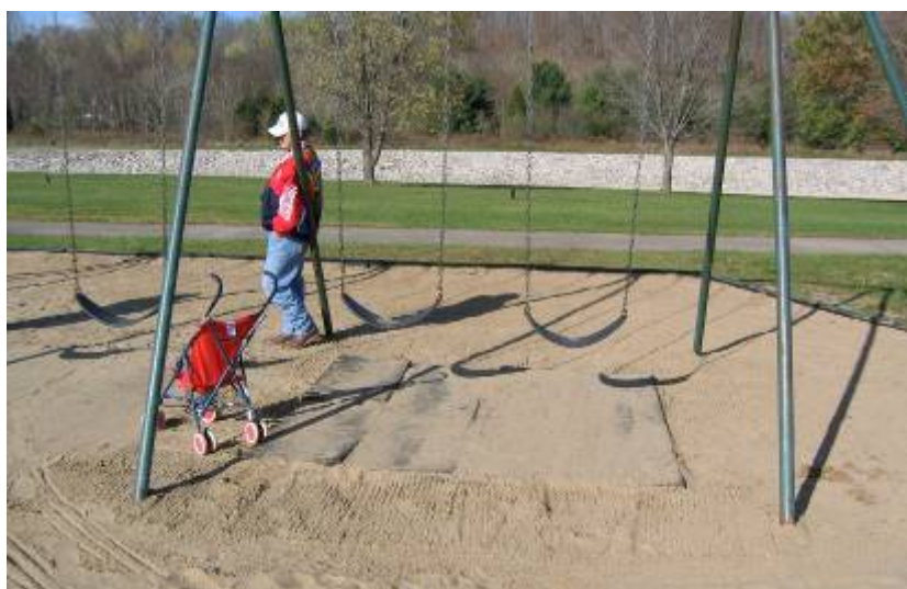
Figure 24. Cave Run Lake, KY. The COE manager uses commercially available rubber pads, buried semi-flush with the ground, to prevent "dips" of compacted soil that hold water directly underneath swings. A specially formulated 2-part glue is used to fasten the pads to a treated wood base that is imbedded in the sand. This installation method keeps the rubber pads in place, and avoids use of metal fasteners that could create a safety hazard
