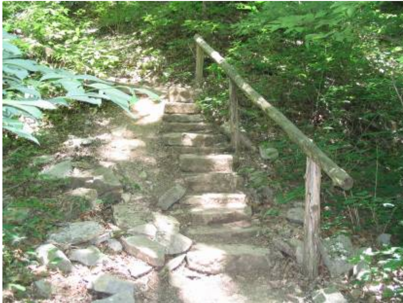
Figure 15. Otter Creek Park, KY. Steps placed on steep sections of trail can prevent erosion problems and provide a safer tread for hikers. This section of trail has steps made from rocks placed approximately seven years ago
