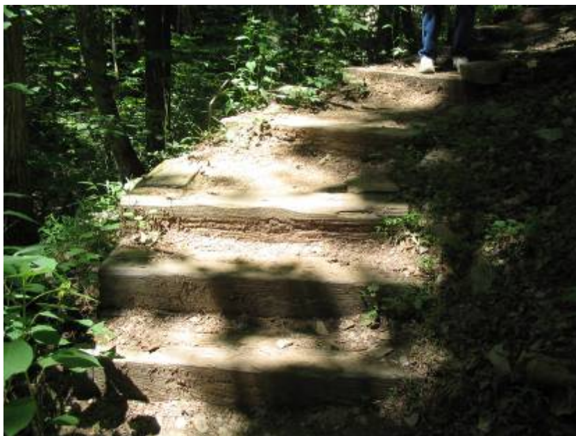
Figure 19. Otter Creek Park, KY. Trail steps made with timbers that have been in place for approximately 15 years. Since this is a dry section of trail and receives some sunlight, the timbers have lasted much longer than a typical five-year life expectancy in shaded, damp conditions
