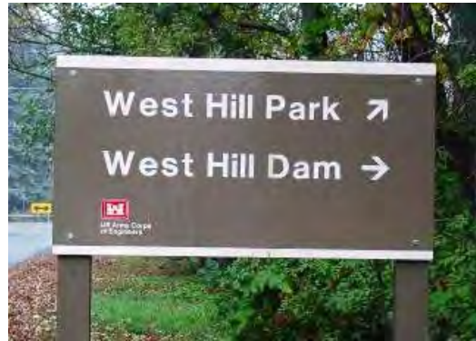
Example of a plywood approach directional (APRDIR) sign.
