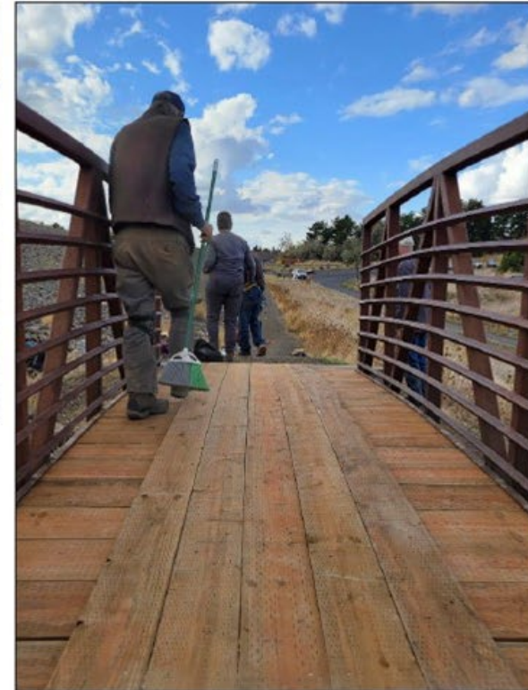
Right: The finished product was a beautiful and durable surface with the center boards taking the brunt of equestrian traffic and being easy to replace without damaging the underlying planks.
