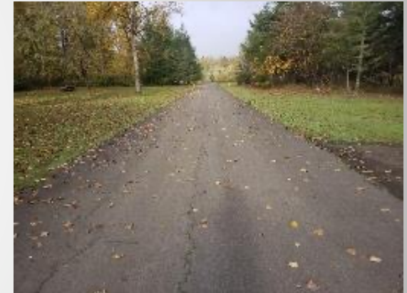
D - HIGH SEVERITY – ALLIGATOR?
