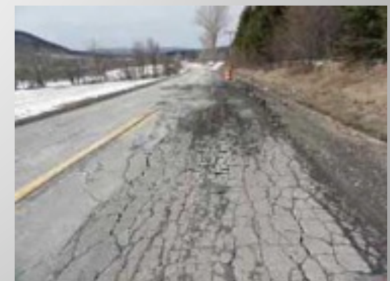
D - HIGH SEVERITY – ALLIGATOR?
