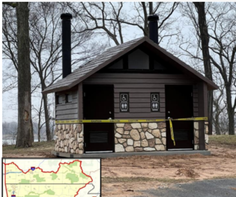
NEW RESTROOM AT DAMSITE 6 PARK
