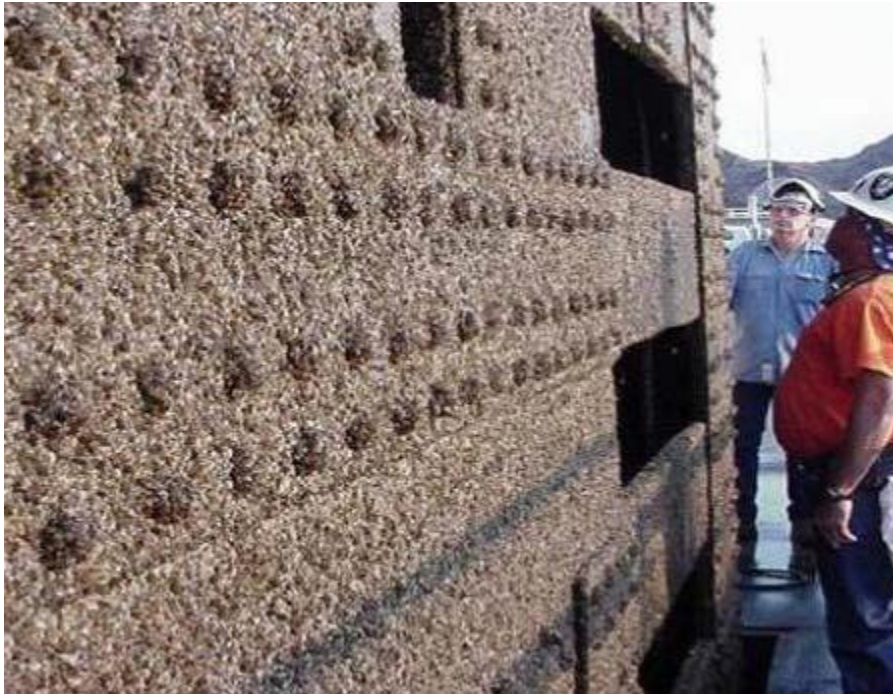
Figure 13. Quagga Mussels on the Davis Dam in California
