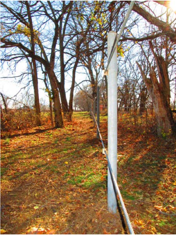
Finished perimeter fence and corrals.
