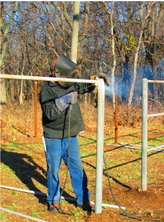
Left: Dale Mitchell welds the top rung of a corral.
