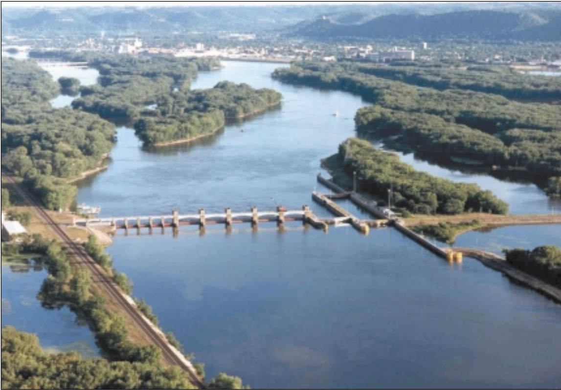
Lock and Dam 5A, Winona, MN. (U.S. Army Corps of Engineers.)
