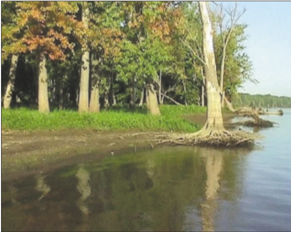
Tree roots exposed by shoreline erosion on the Upper Mississippi River. (U.S. Army Corps of Engineers.)
