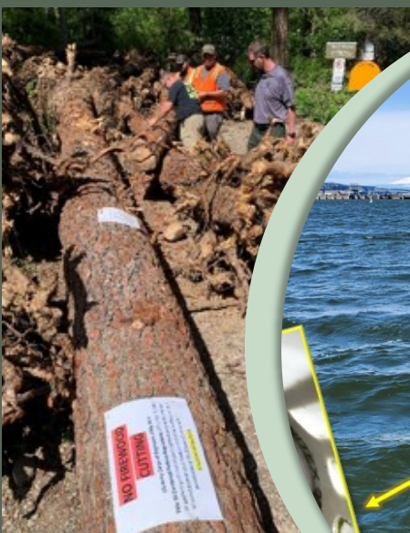
Photo Upper Left: Conducting the first round of placement at Alexander Creek. Photo Lower Left and Right: Collecting logs at burn piles. ID tags are being used to track wood in the river as part of the monitoring phase of the project.
