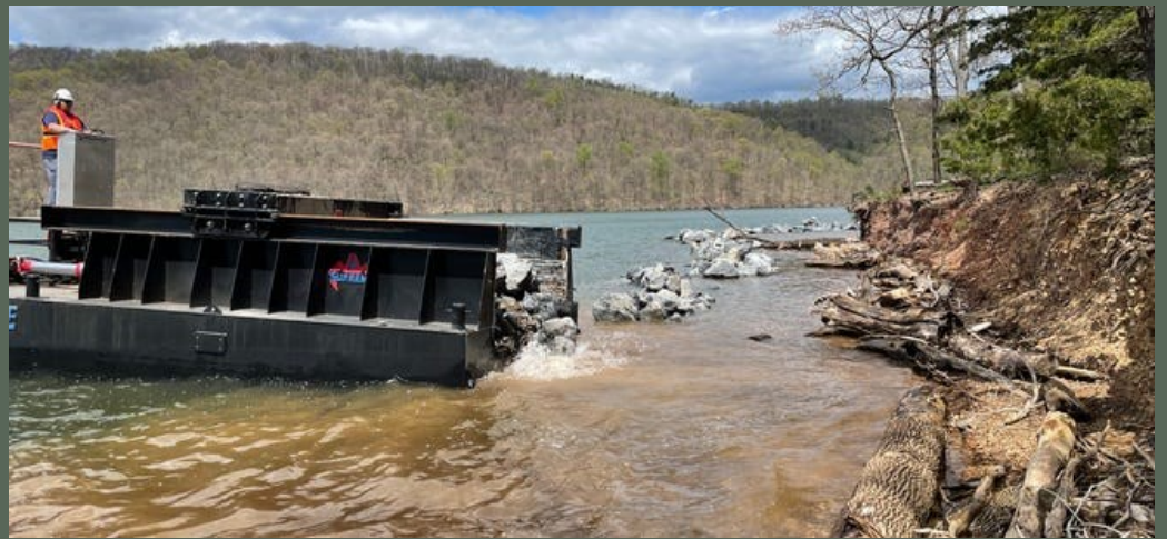
Photo above: Crews unload rocks along the shoreline of Raystown Lake to create better fishing habitat and reduce shoreline erosion. Photo provided by Ben Page, PAFBC.
