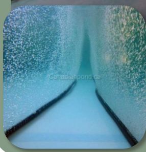
Photo Above: Pictures of bubble curtain post dye treatment to determine water exchange rate. Photos Left and Right: Pictures from manufacturer Canadianpond.ca of the bubble curtain.
