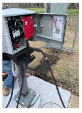
The site will receive three Ford F150 Lightning trucks later this month, which are estimated to take 10 hours to fully charge using the installed Level 2 chargers. Overnight recharging should not be an issue, especially as typical daily use will not fully deplete vehicle charge. Additional EVSE on the FY22 MATOC are expected to be installed over the coming months, so stay tuned!
