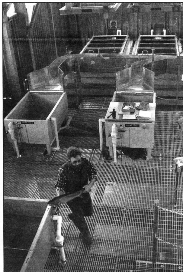
A new fish trap system at Lower Granite Lock and Dam tripled the system's tank capacity, giving researchers easier handling of migrating adult salmon and steelhead. (Photo courtesy of Walla Walla District)
