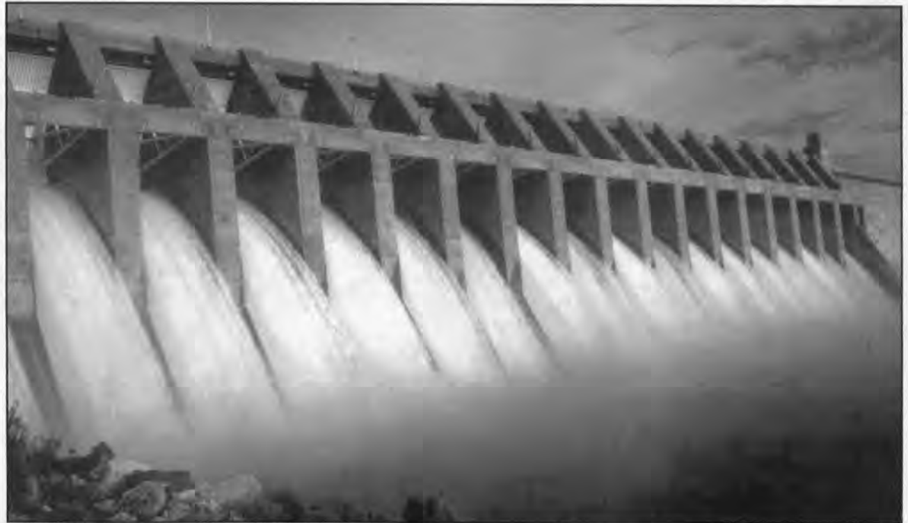
Flow deflectors installed at Chief Joseph Dam are preventing damage to fish due to high-pressure gas forced into the water. (Photo from the Digital Visual Library)
