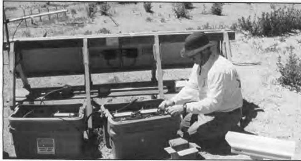
John Gagnon hooks up batteries and a solar panel to power web-cams to monitor nesting sites. (Photo courtesy of CRREL)
