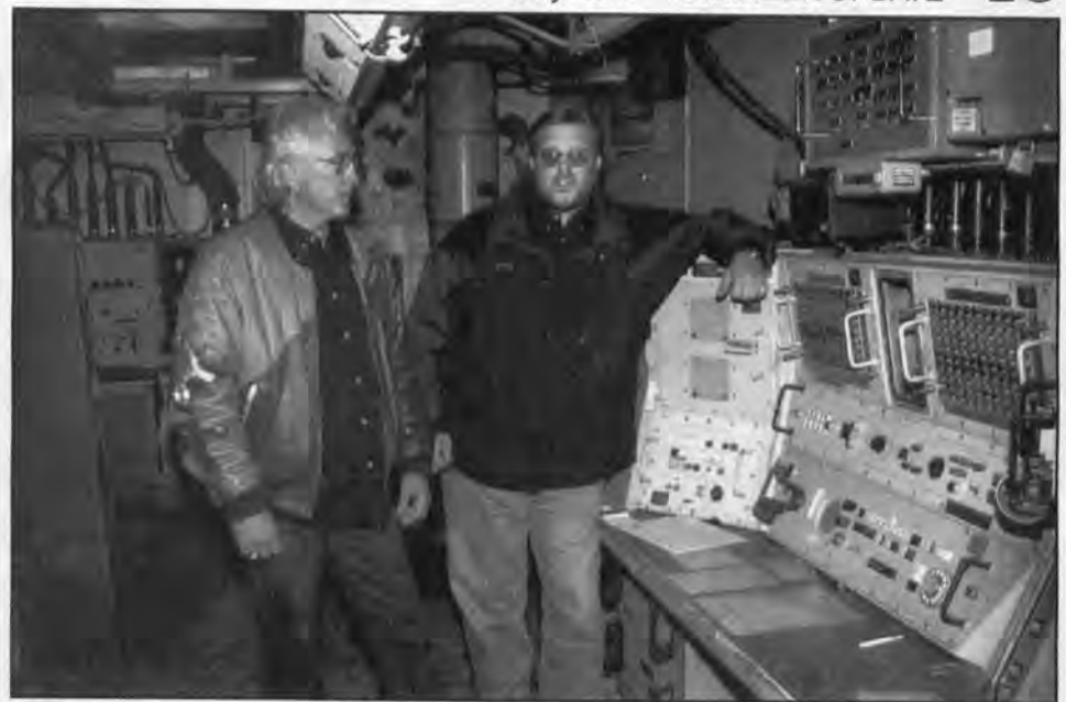
Vaughn Viet (left) and Bart Anderson, both contractors, stand in the control room of an old Minuteman missile silo. Anderson is leaning on the launch control panel. The control room will be welded shut, and the elevator shaft filled with debris. (Photo courtesy of Omaha District)
