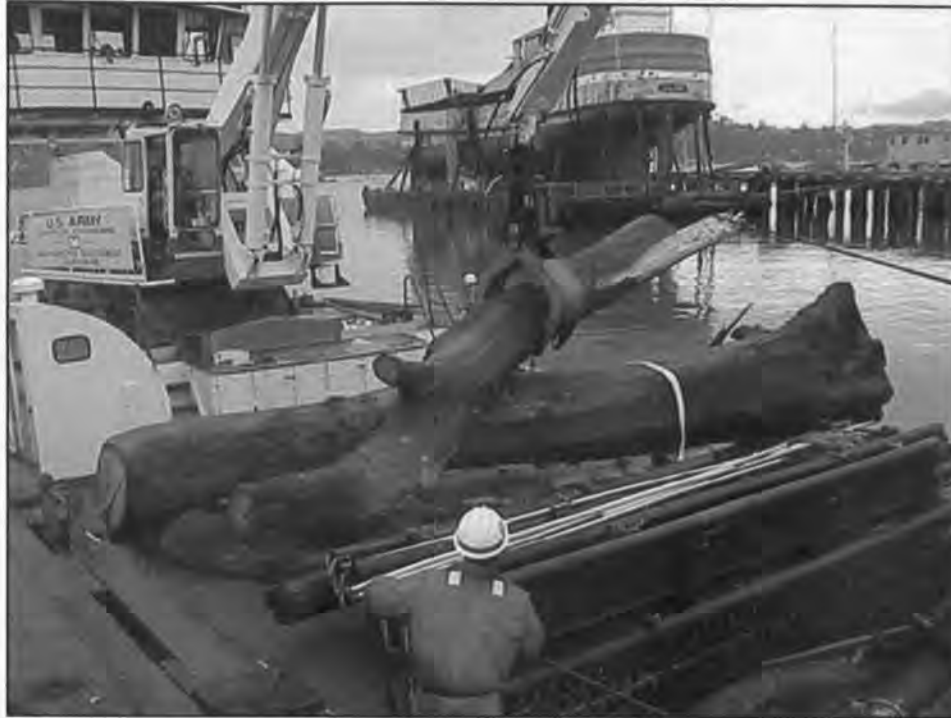
Debris collection in San Francisco Bay is one of San Francisco District's high-visibility civil works missions. Crews collect about 80 tons of debris a month. (Photo courtesy of San Francisco District)
