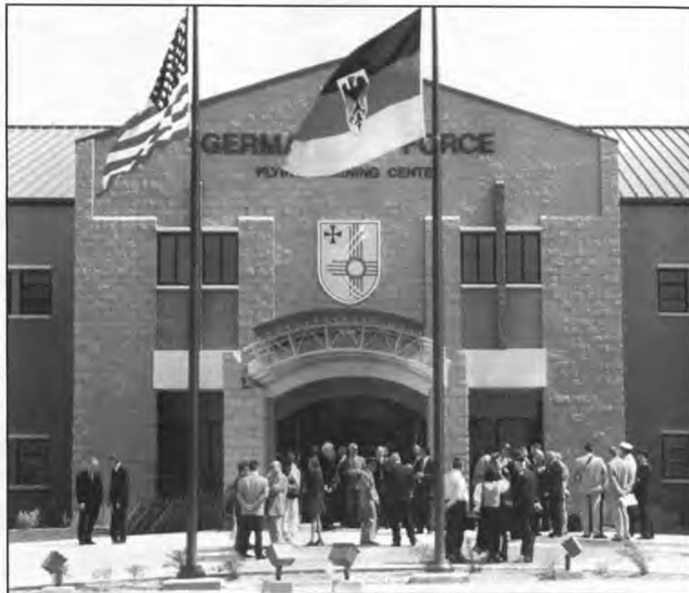
Albuquerque District manages $100 million in construction to support the German air force's Tornado beddown program at Holloman Air Force Base, N.M. (Photo courtesy of Albuquerque District)
