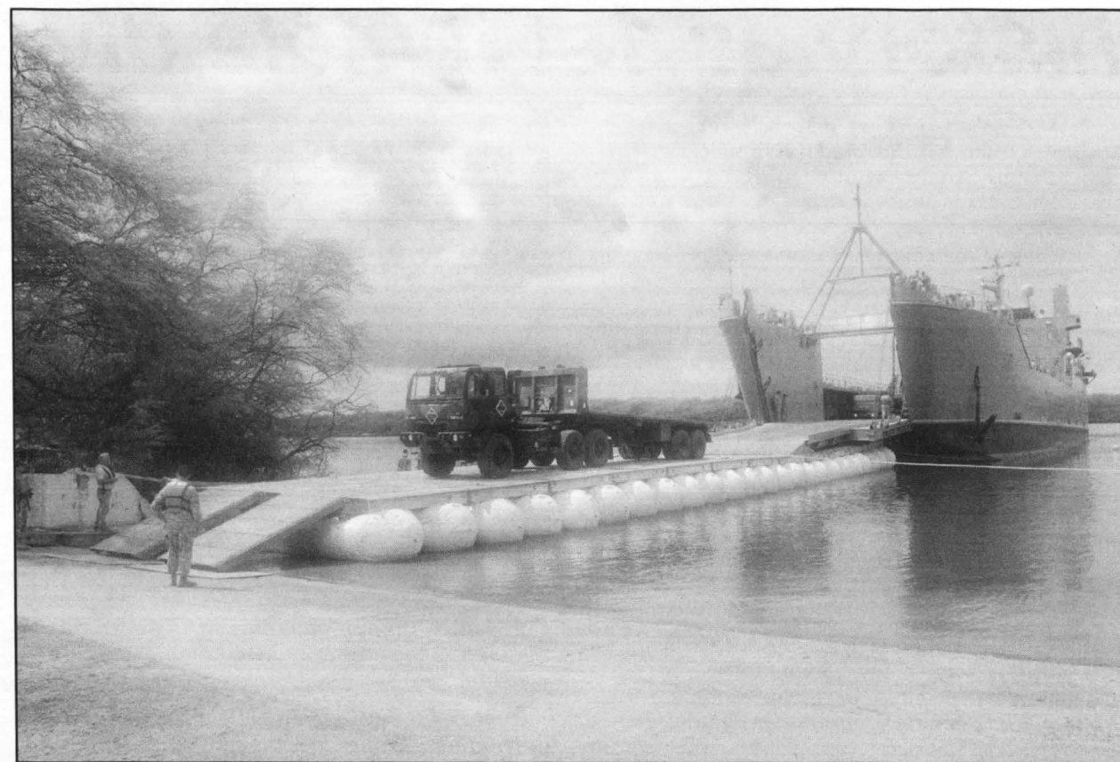
ERDC's lightweight modular causeway system was successfully field demonstrated last September. (Photo courtesy of ERDC)
