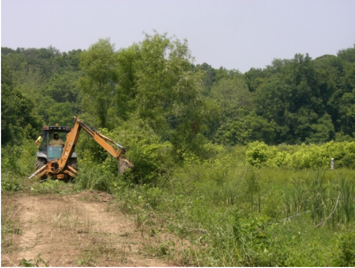
Ohio Department of Transportation heavy equipment operators started by clearing the vegetation from the dam (left). The finished dam and wetland (right) immediately started to attract wildlife including a startled white-tailed deer (below).
