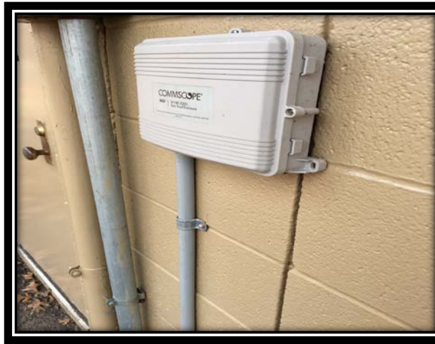
Fiber Optic Termination On Building
