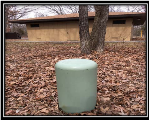
Fiber Optic Cable Splice
