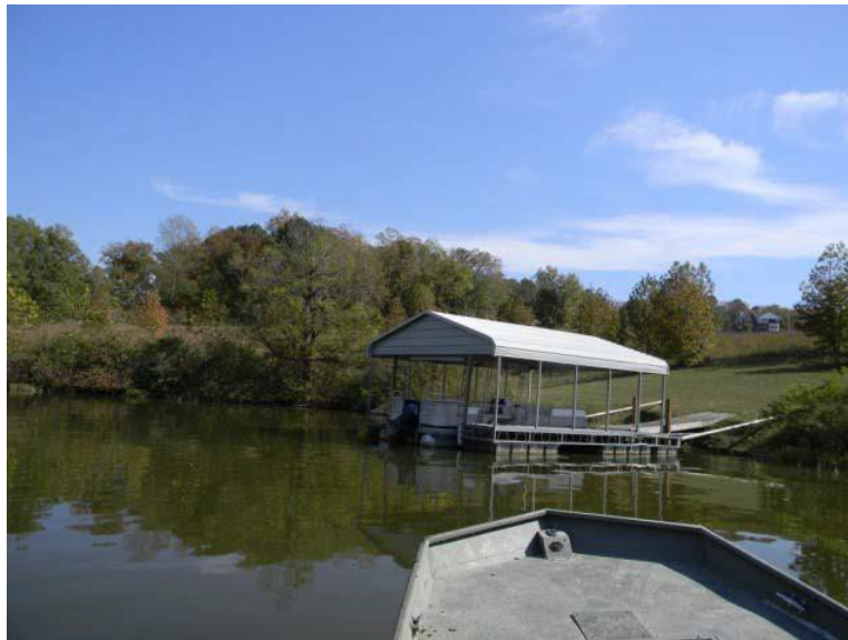
Regular dock permit inspections are conducted at lakes which have shoreline management programs.
