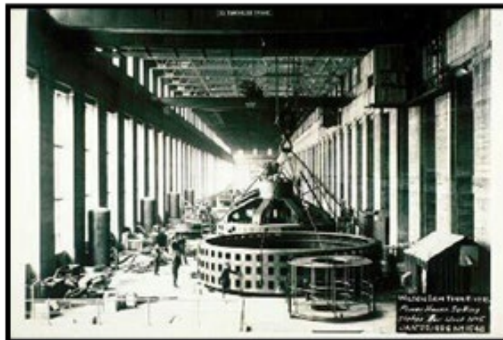
Wilson Powerplant, Florence Alabama, ca. 1926. Constructed by the Corps of Engineers.
