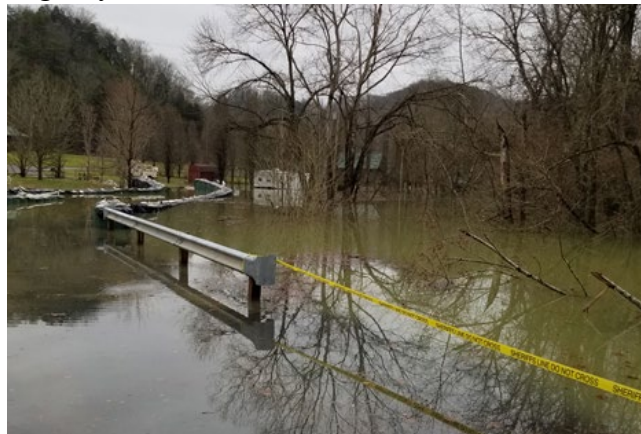
Flooding below Wolf Creek Dam during 2019 high water event
