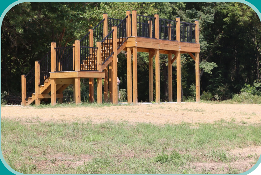
Elevated archery shooting platform
