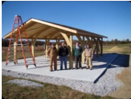
Hannibal Career & Technical Center faculty complete construction
