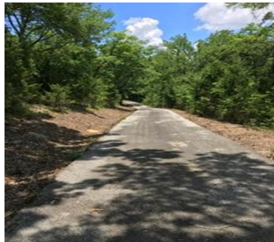
New Trail at Hurricane Bridge
