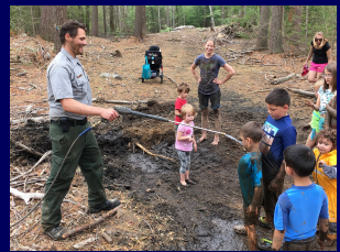
Ranger Ron Woodall uses a pressure washer and 100 gallon truck-mounted water tank to aid in clean up
