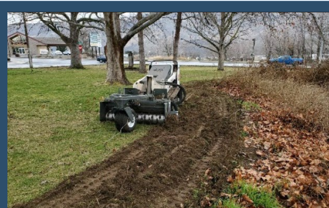
Photo: Front view of a minicat with soil conditioner attachment that was used to prep the site for planting.
