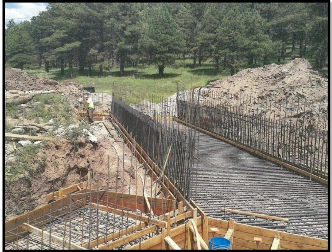
Concrete box culvert – view to Northwest
