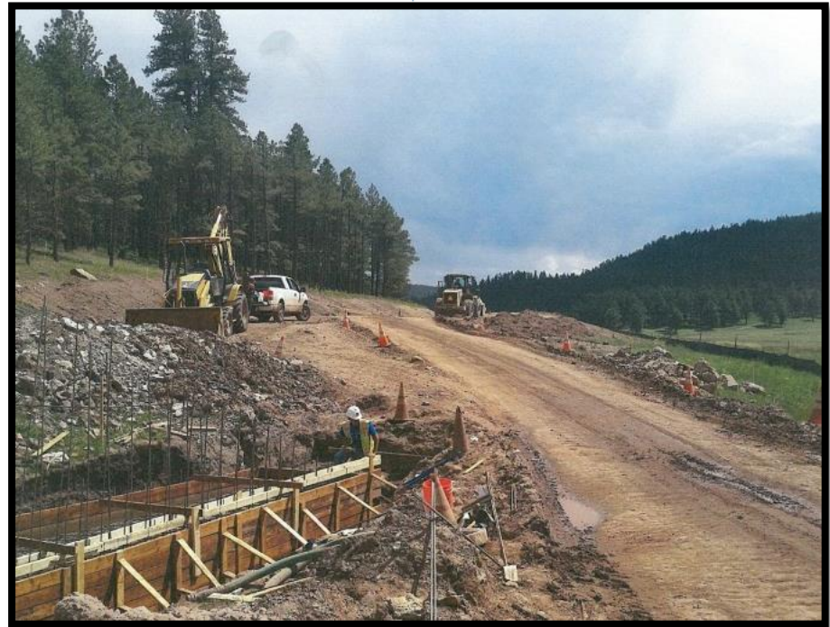
Roadway subgrade preparation – view to Southeast
