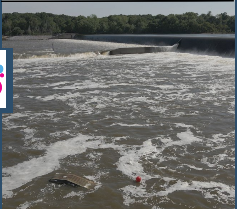
Photo 4: A surplus vessel was used to create a water safety video on the hazards of a fixed crest spillway. The sUAS was able to capture shots from locations that were unsafe for personnel.
