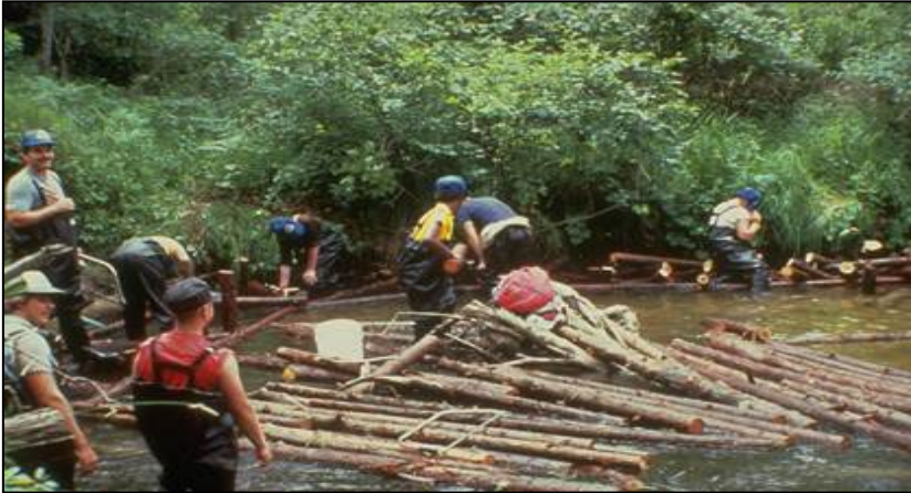
Pre-1990's: Local, in-stream projects
