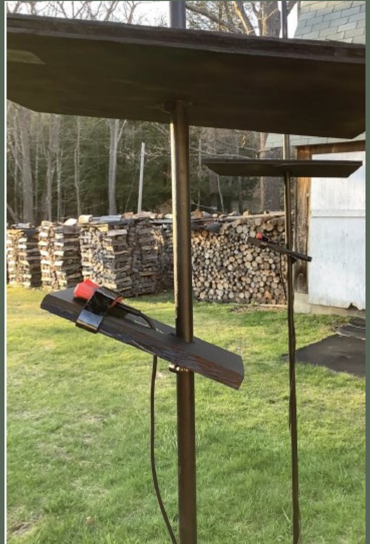
Photo: Example of an acoustic monitoring system deployed at the Edward MacDowell Dam. Photo provided by Dr. Jacques Veilleux, Ph.D., Franklin Pierce University.
